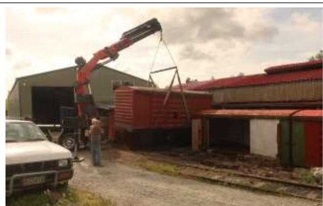
First - lay concrete further along from old KP (freight wagons); then lift the KPs & move them out of the way using flat wheeled wagons
