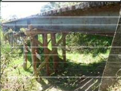
Temporary piling work has been carried out on pier one of Longbridge . This will enable the engines only to enter clear of the points as they run around for our passenger rains .
