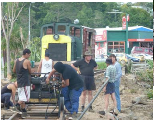
(Above) Mike and Malcolm tidying up the embankment (Below) The relaying and spiking of the sleepers begin.
