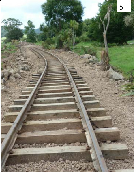
(Above) All the sleepers and spikes are back in place and await ballasting. (Below) Graham Winterbourn lays the ballast as the ballast wagons come into service for the first time
