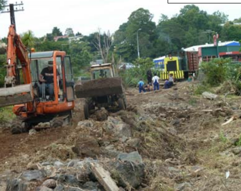
Below Work starts on restoring the embankment
